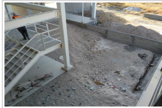
F5: Vista al interior
